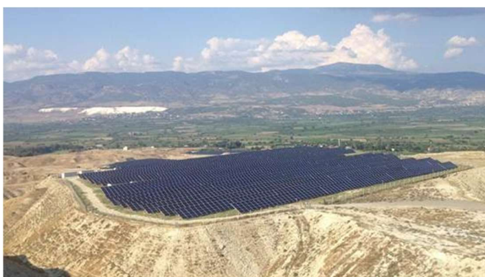
Solar power plant in Denizli Province, Republic of Turkey Power generation capacity 13.514 MW
