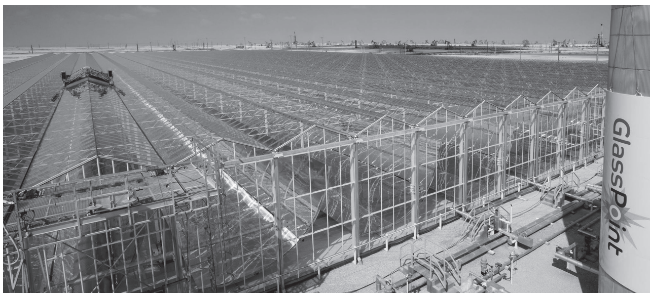
Mirraah Solar Park: One of the world's largest solar parks. Miraah (meaning mirror in Arabic) is a 1,021 MW solar thermal facility in South Oman, harnessing the sun's rays to produce steam for injection into an Omani oil field.
